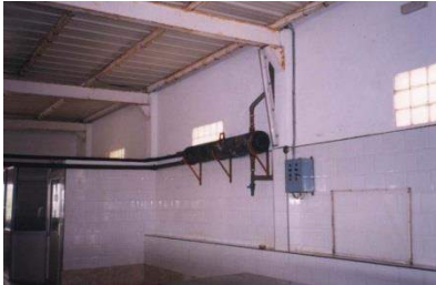
UV sterilizer in oyster hatchery - Morocco
