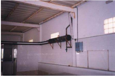
UV sterilizer in oyster hatchery - Morocco
