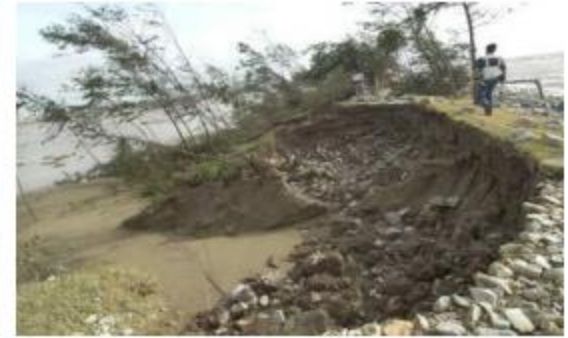
Sea dike erosion at Nam Dinh coast during typhoon
