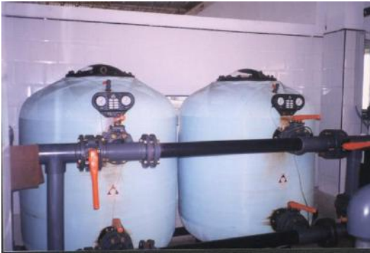
Sand filter – oyster hatchery Morocco
