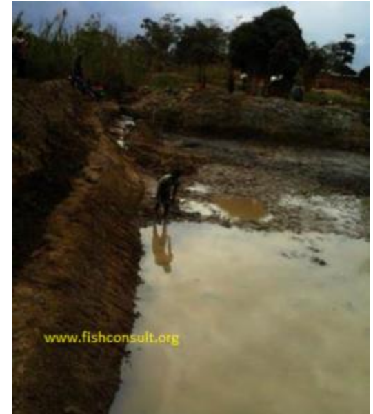
Construction of communal fish ponds in Songea
